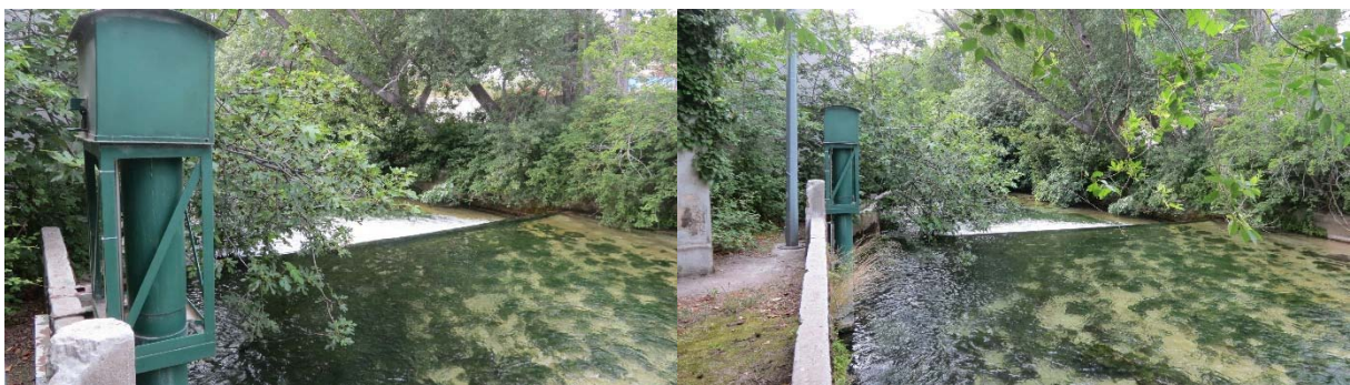
Hydrological gauging station downstream of water intake structure
